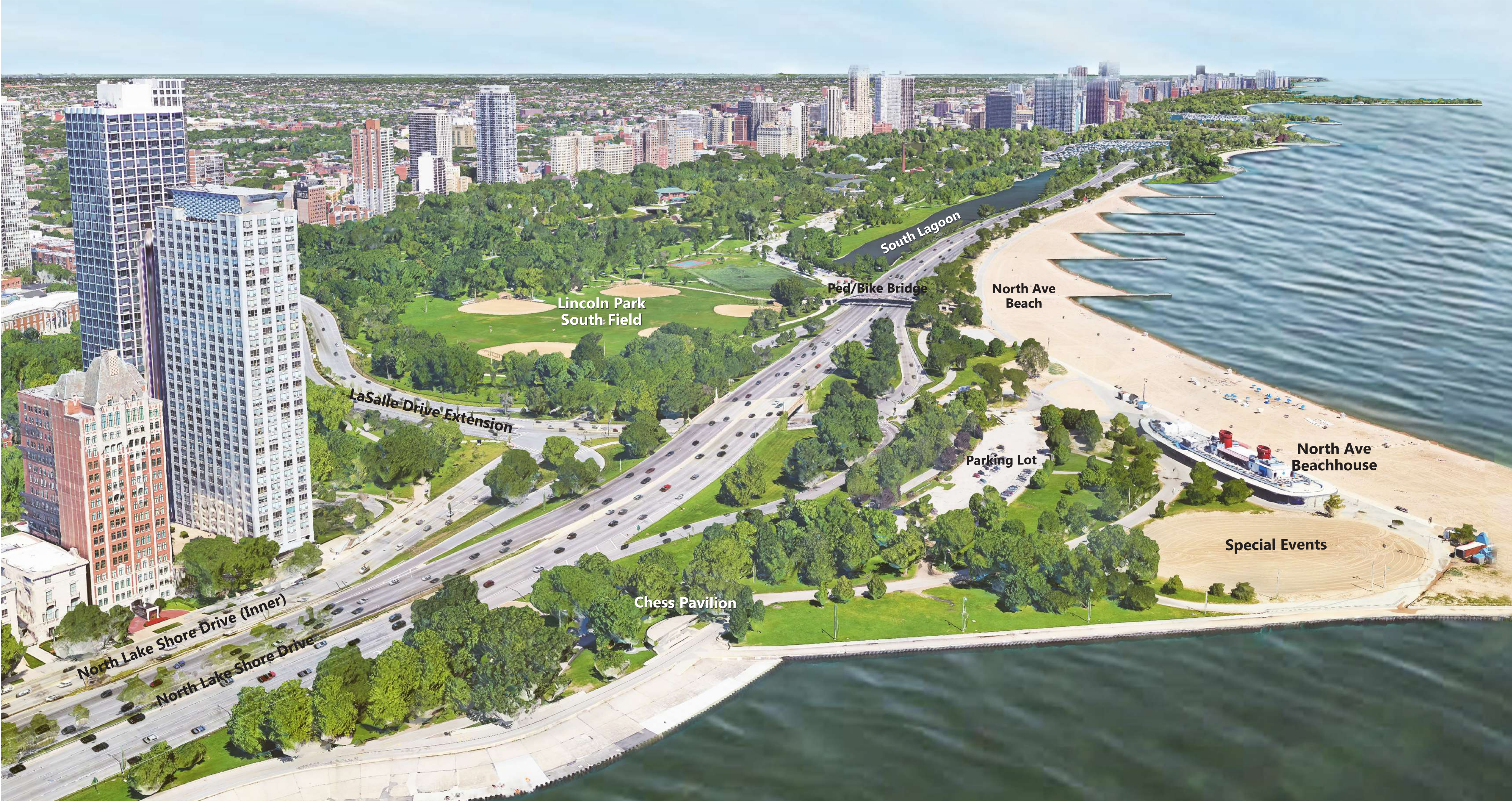
LaSalle Drive Looking North - EXISTING VIEW
